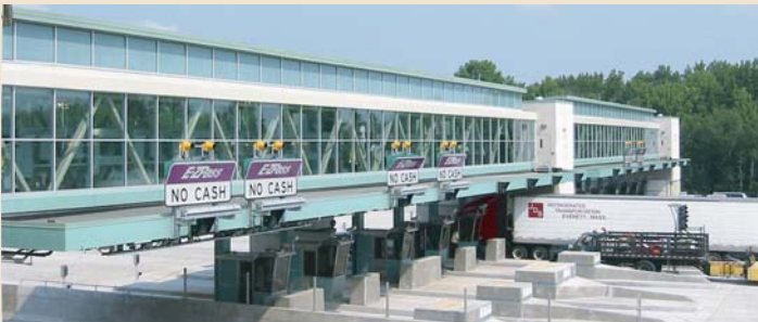
Construction Inspection Services for Interchange No.1- NJTA
