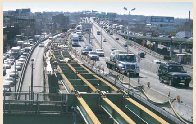
Construction Inspection for Emergency Repairs along the Gowanus Expressway Viaduct (I-287), Kings County, NY - NYS DOT
