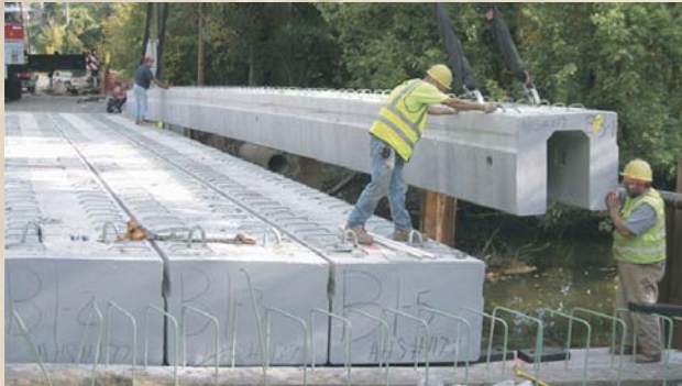
Replacement of Troy Road Bridge over Whippany River, Construction Inspection East Hanover Morris County, NJ
