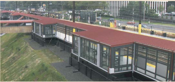
Construction Management Services for Metropark Station Platform Reconstruction-NJ Transit
