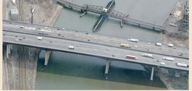
Construction Inspection Services for Bridge Deck Reconstruction and Miscellaneous Structural and Roadway Improvements, over Passaic River - NJTA
