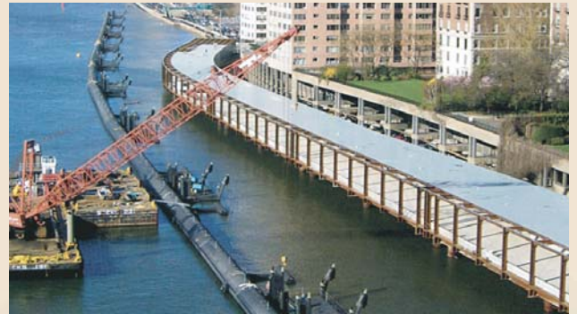
Construction Inspection for FDR Drive SB (E.56 th to E.64 th St.) Reconstruction - NYSDOT
